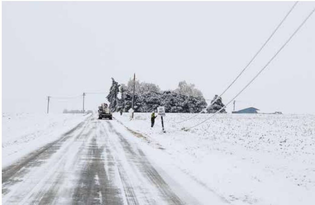
causing the lines to touch or rest on one another. Because of this, melting ice can cause outages even though the temperature is rising. Depending on conditions, melting ice can cause as many or more problems than the ice itself.
